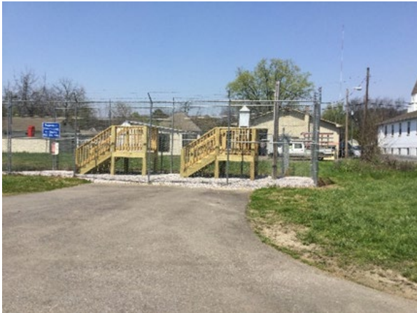
Figure 3.5 Ameristeel Site View
