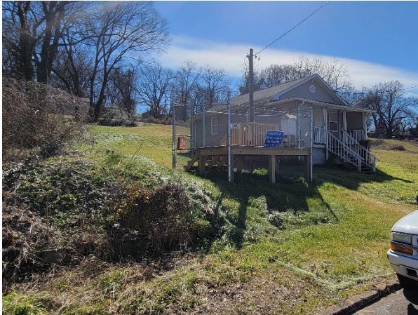
Figure 3.13 Parton Place Site View
