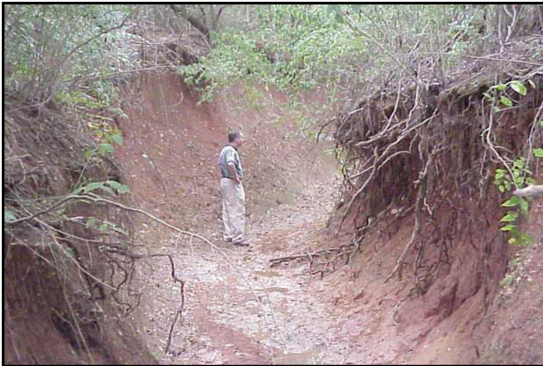
Figure 2-2. Example of Significant Streambank Erosion
